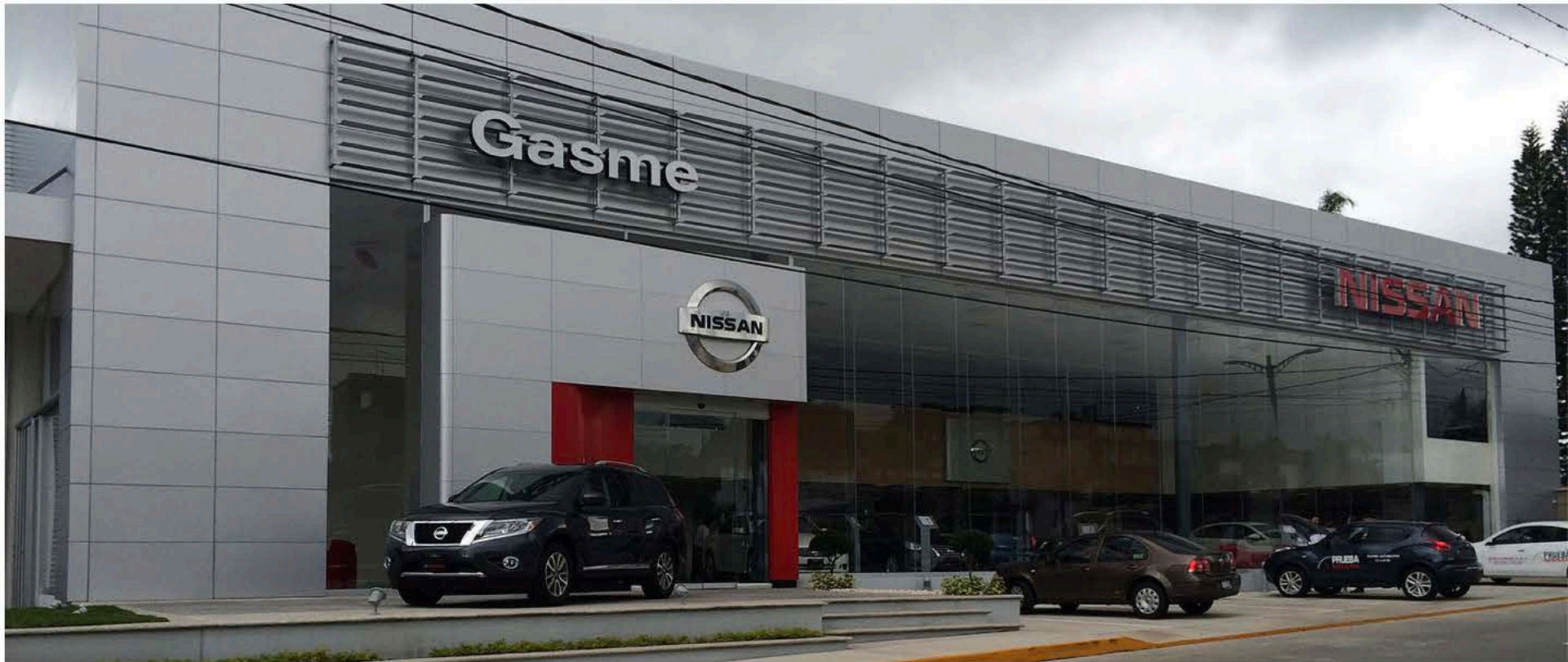
Nissan Gasme Cordoba, Ver. Glass Facade Clear Temp 3/8" 4,975 sqft Gilca Constructora
