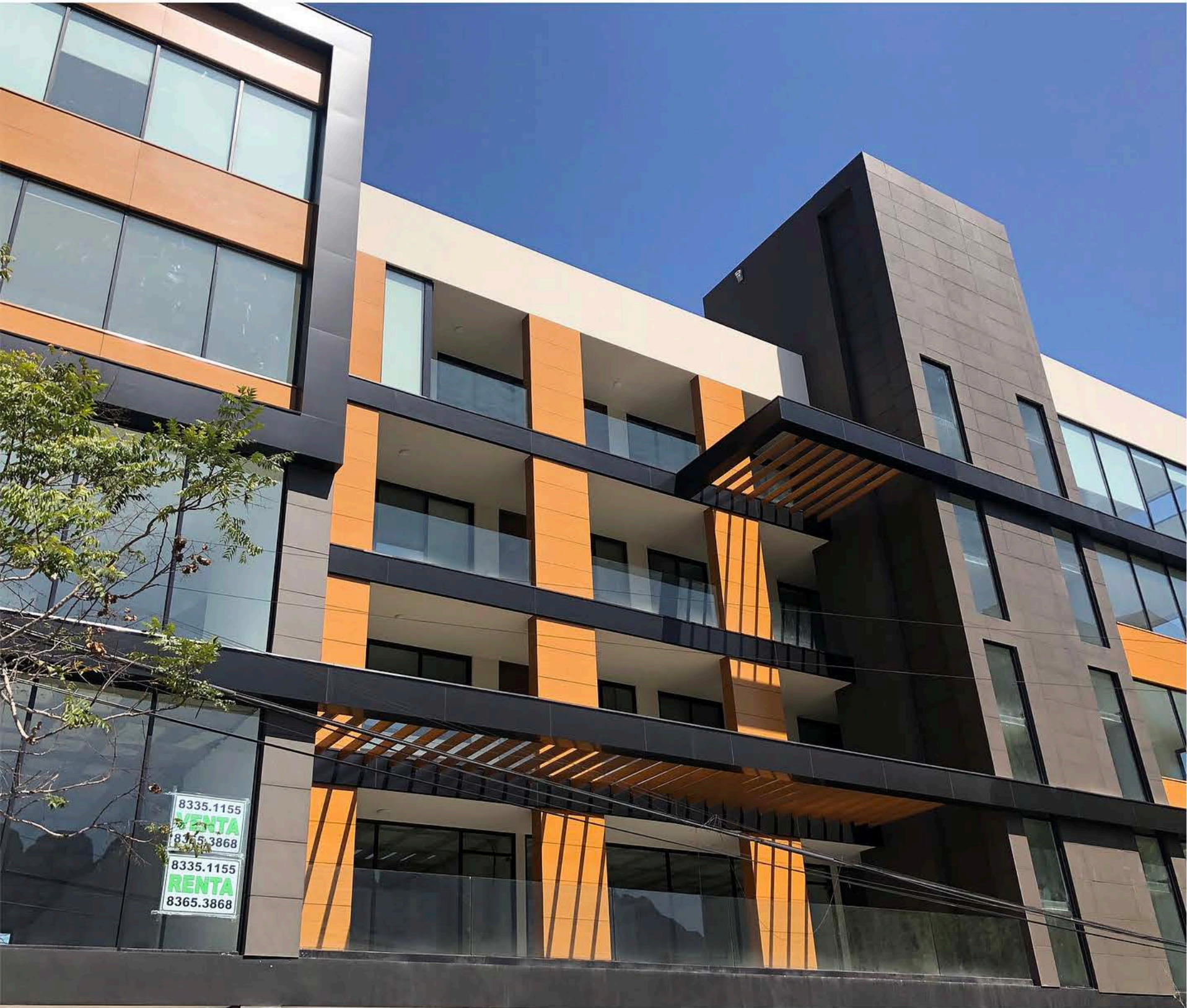
Guadalquivir I Apartments Del Valle, Garza Garcia, N.L. Cuprum C 140, C 70 & C 50 Insulated Clear Temp ¼” + Clear Temp ¼” 5,937 sqft Trecasa
